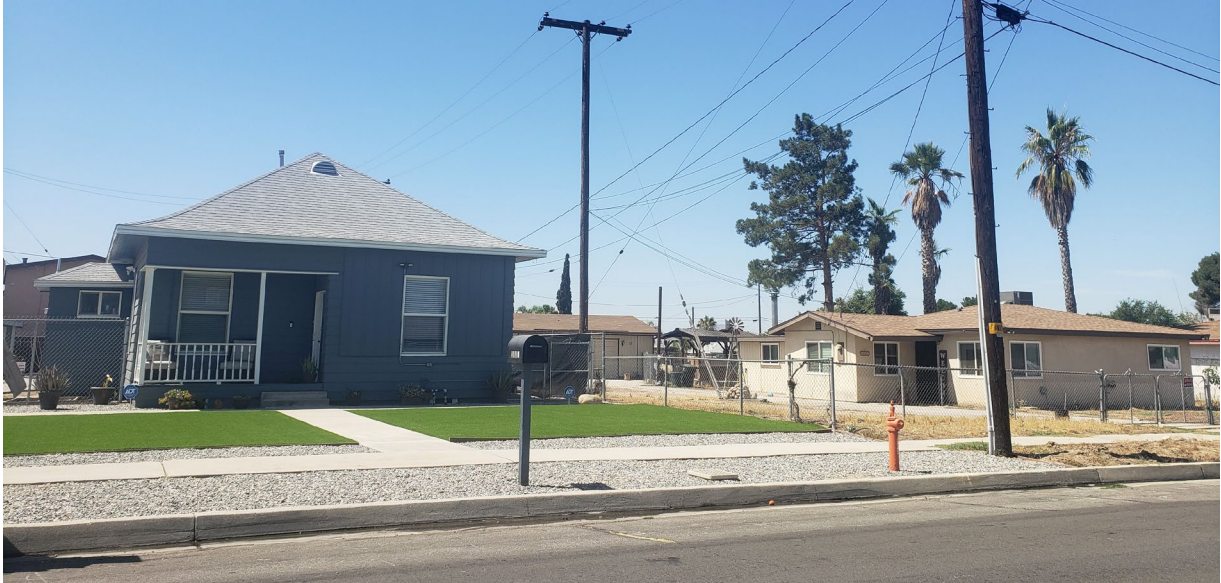
Homes that would be demolished for the Airport Gateway Project. Photo credit: Economic Roundtable.
